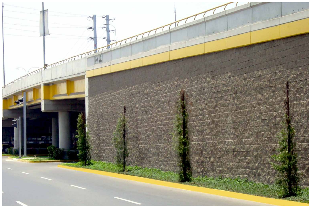
▶ Earth reinforcement walls
