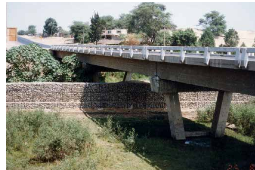
► Bridge abutment protection
