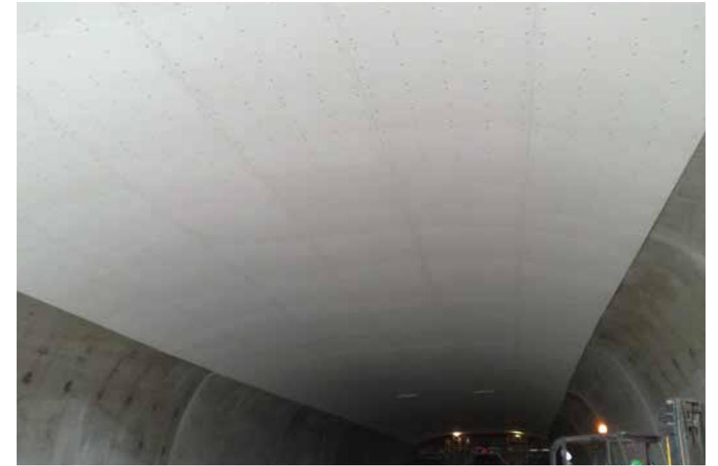
► Tunnel fire-proofing
