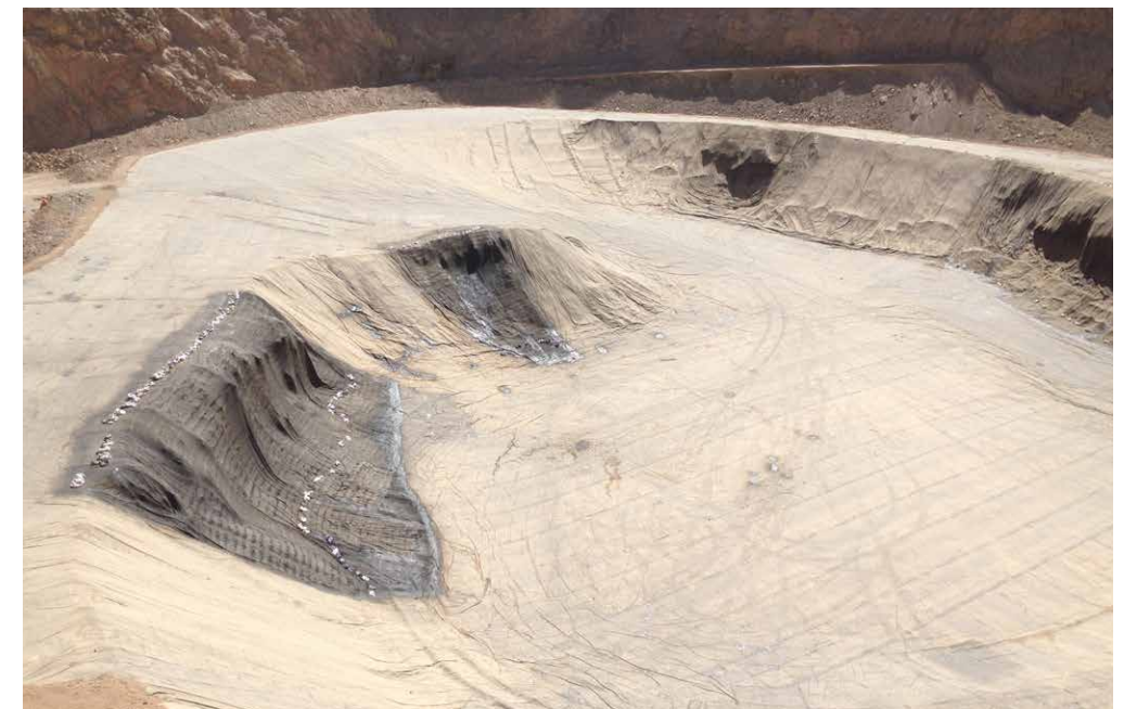
► Liquid waterproofing - Mantos Copper, Chile
