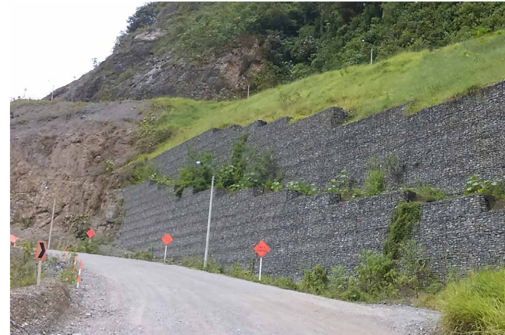
▶ Mechanically stabilized earth walls
