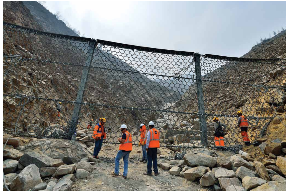
▶ Rockfall protection and natural hazards protection
