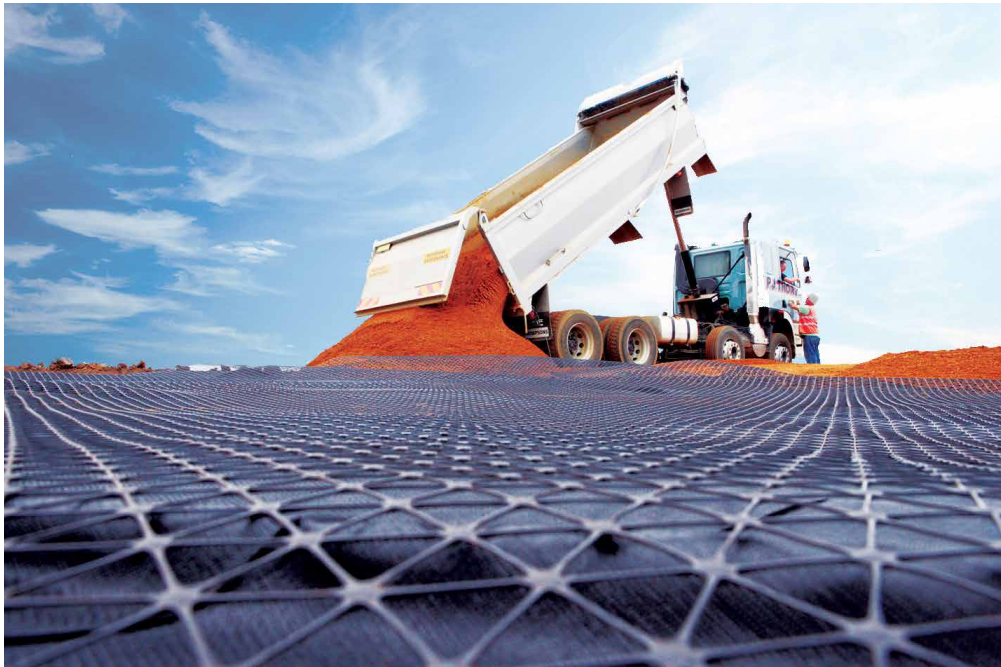
► Road stabilization and reinforcement
