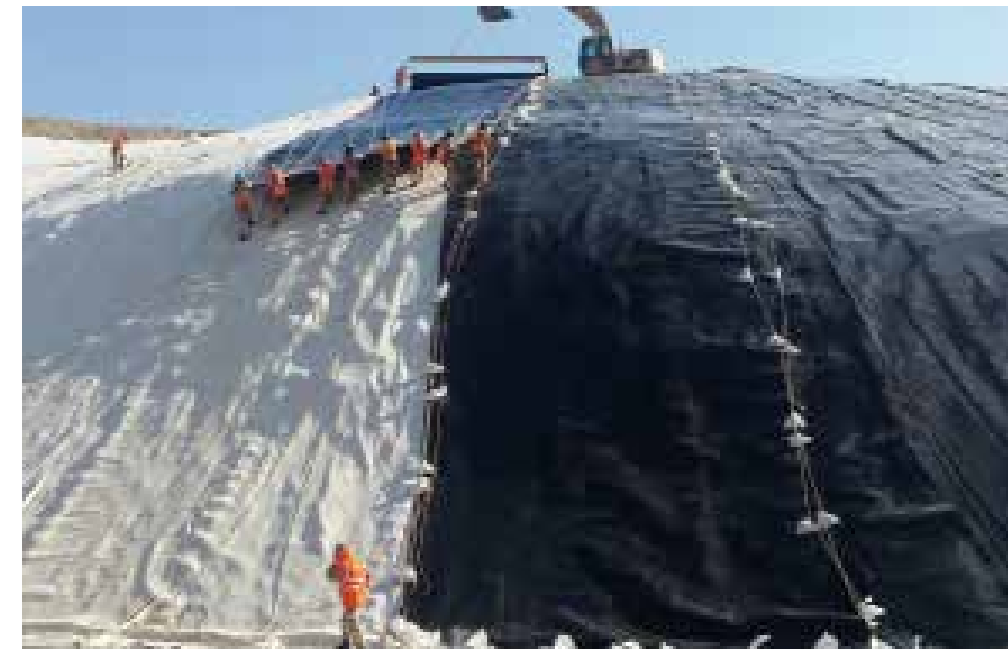
► Geosynthetics installation
